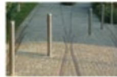
Railway segments inserted into the paving
